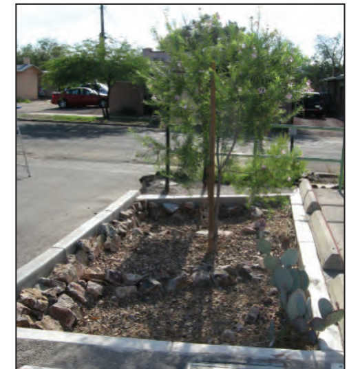
Figure 4-32 Bioretention cell installed as retrofit, Tucson AZ. Note flush curb on three sides and surface graded against low curb wall to retain stormwater. Photo courtesy of Watershed Management Group. http://www.watershedmg.org/green-streets
