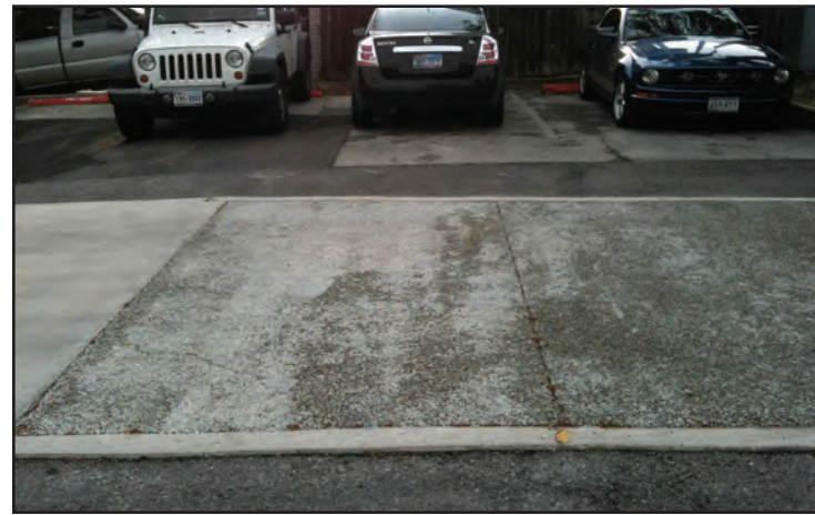
Figure 4-35 Porous concrete pavement installed at Alamo Heights Fire Station.
