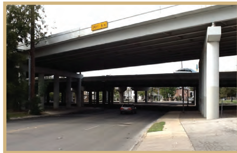
Flores Street Underpass at Interstate 35
