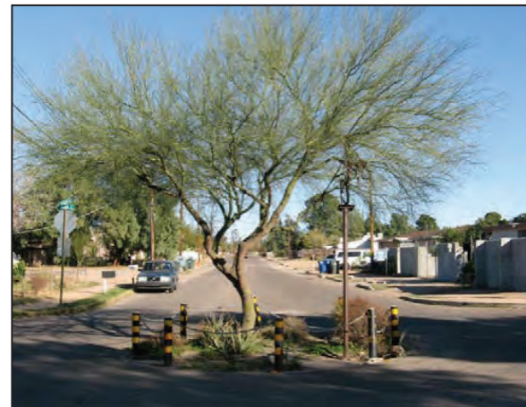
Figure 4-39 Traffic circle used to capture street runoff, Tucson AZ. Photo and text courtesy of Watershed Management Group. http://www.watershedmg.org/green-streets
