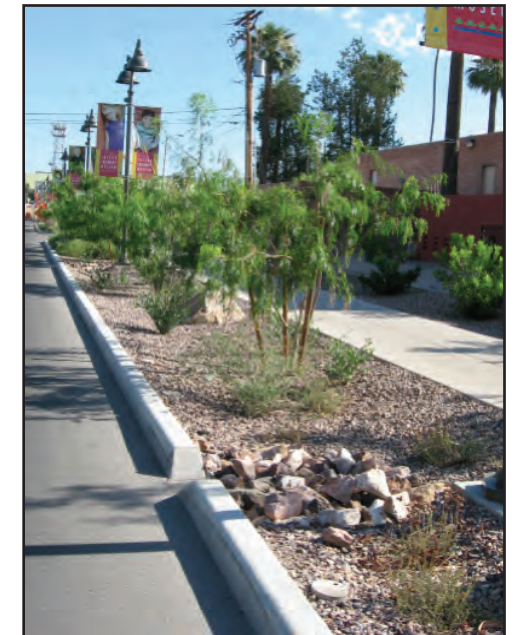
Figure 4-31 Bioswale installed in Tucson, AZ. Photo courtesy of Watershed Management Group. From Green Infrastructure for Southwestern Neighborhoods. http://www.watershedmg.org/green-streets
