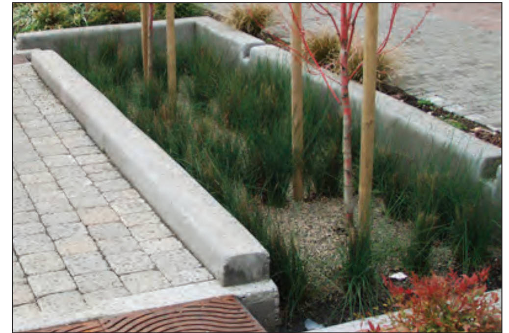
Figure 4-38 Stormwater planter, Portland OR. Source: http://www.phillywatersheds.org/what_were_doing/green_infrastructure/tools
