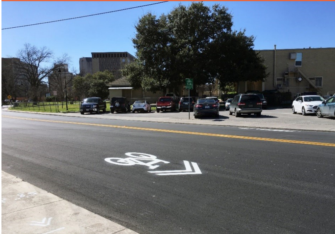
Sharrow marking on St. Mary's Street, San Antonio, TX.
