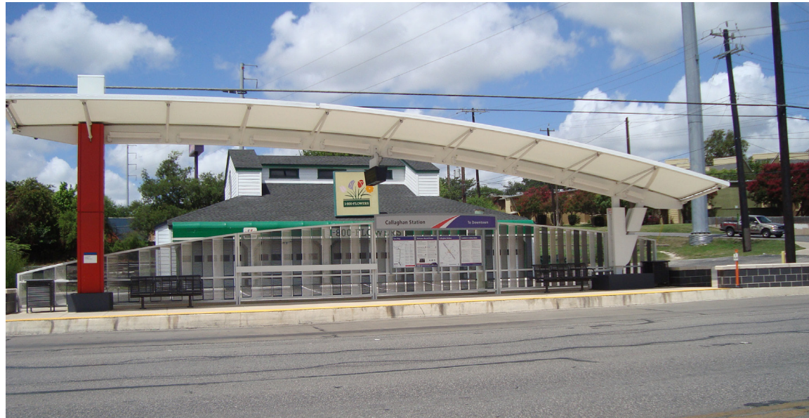
VIA Primo Station along Fredericksburg Road
