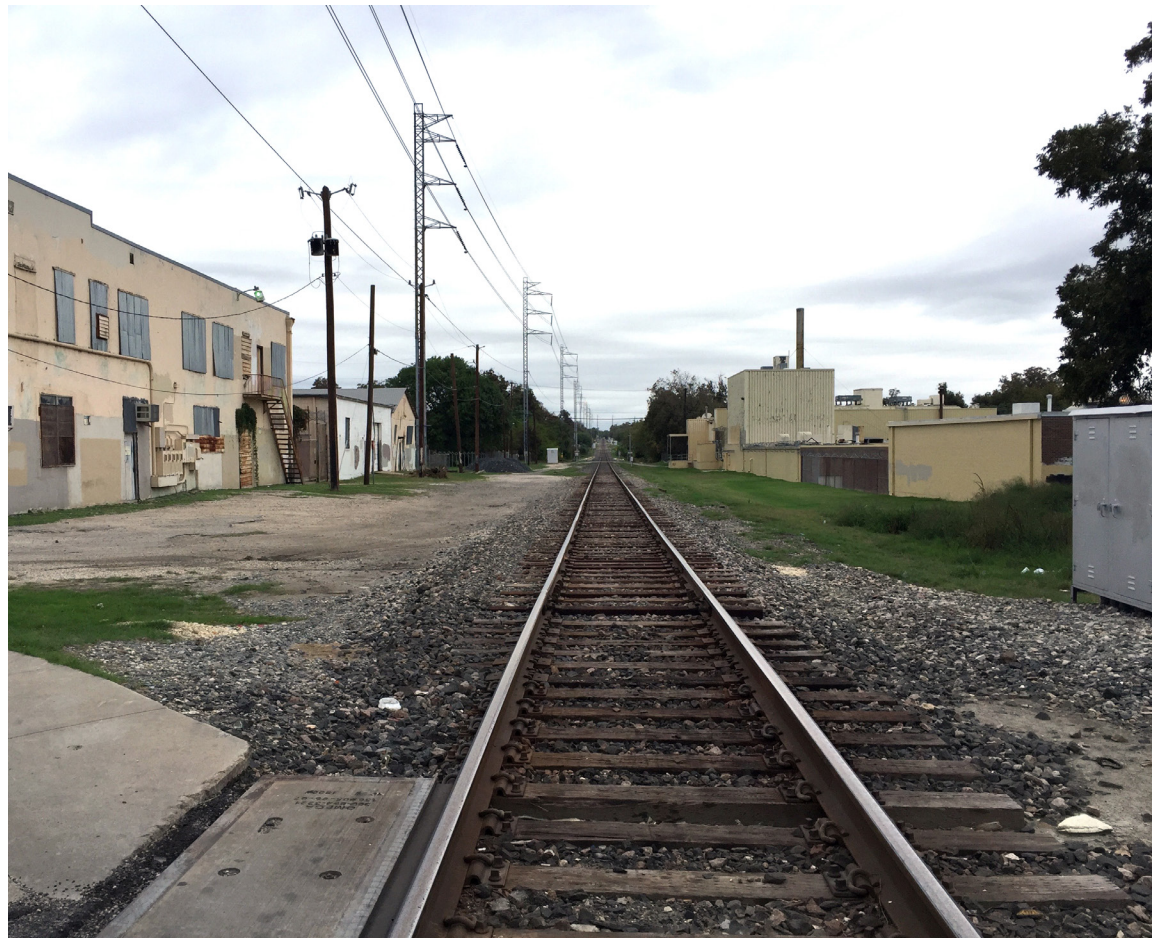
Grade Crossing on Fredericksburg Road, South of Myrtle Street, San Antonio, TX
