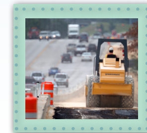
Freeway Widening $7.2 million per lane mile
