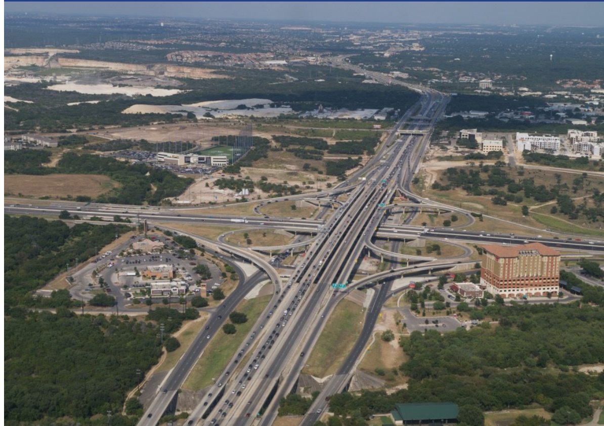
Loop 1604 and IH-10 Interchange
