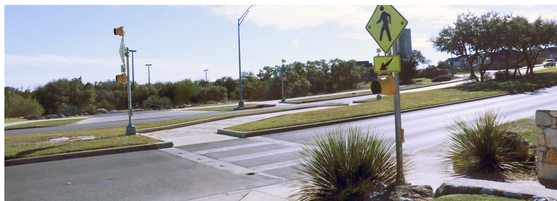
Midblock Z-Crossing With Runway Lighting And Flasher On Stone Oak Parkway
