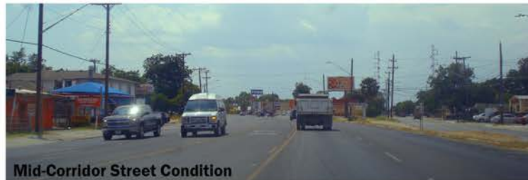
Mid-Corridor Street Condition
