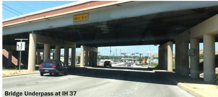
Bridge Underpass at IH 37
